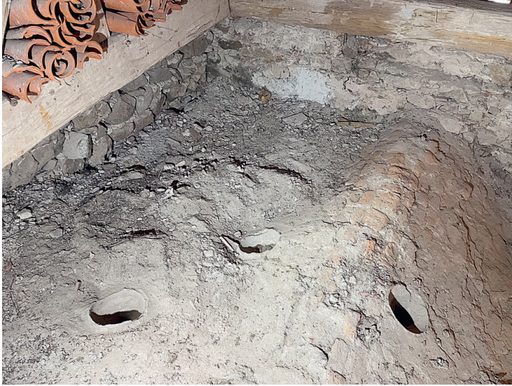
Fig. 4. Church of St. Gall in Myšeneč, attic, brick vault of choir with embedded vessels (photo by F. Facincani).
