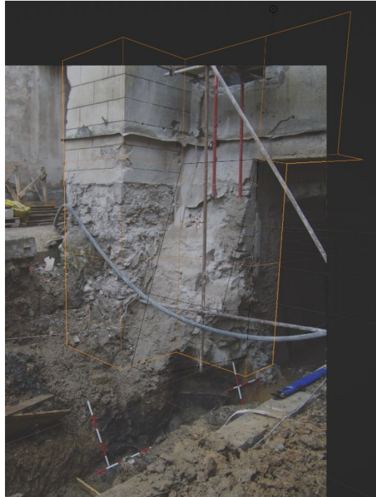
Fig.3 Control of angles, dimensions, and deformations through the fSPY add-on in Blender.
